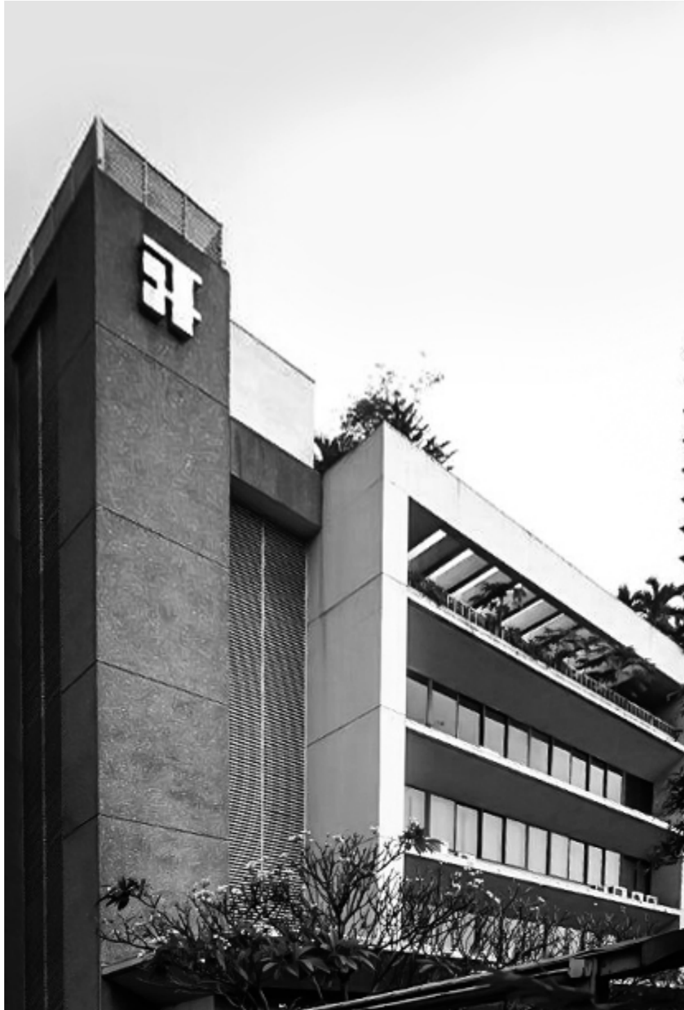
GF & Partners Building along HV Dela Costa Street, Makati City. The old GFP office was one of Ar. Formoso's last projects before his retirement.
